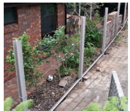
Set all the bottom rails into position ensuring a 50mm ground clearance.
