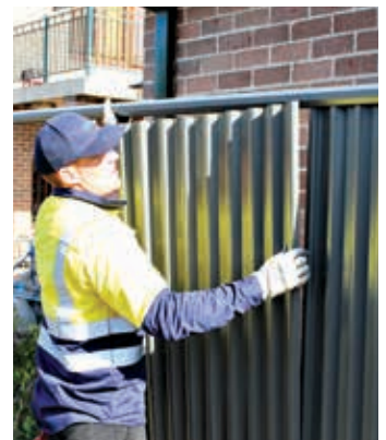
Place 2nd & 3rd sheets into bottom rail, ensuring there is sufficient overlap.
